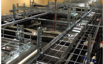
Our unique beam clamp system offers limitless combinations. We have solutions and equipment for building your own 19" rack. Accessories like horizontal and vertical cable trays give you an open rack with ample working space and free passage for cooling air. All the system parts are compatible with each other and it is easy to screw the installation together into one unit.
